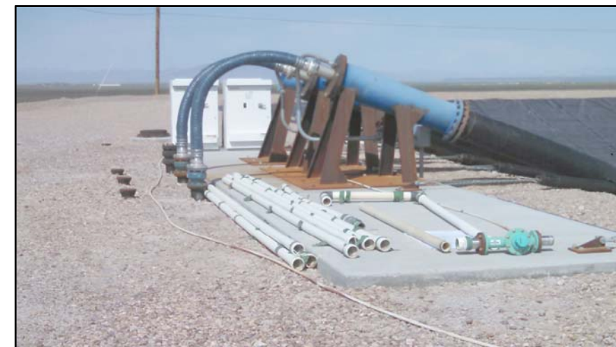
EXISTING BRINE RECOVERY ANCHOR SYSTEM FROM SAWTOOTH BRINE POND 1 FOR FABRICATION REFERENCE
